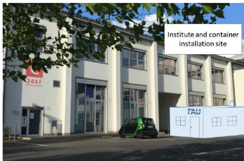
FAU lab and envisaged installation location of the pilot building
